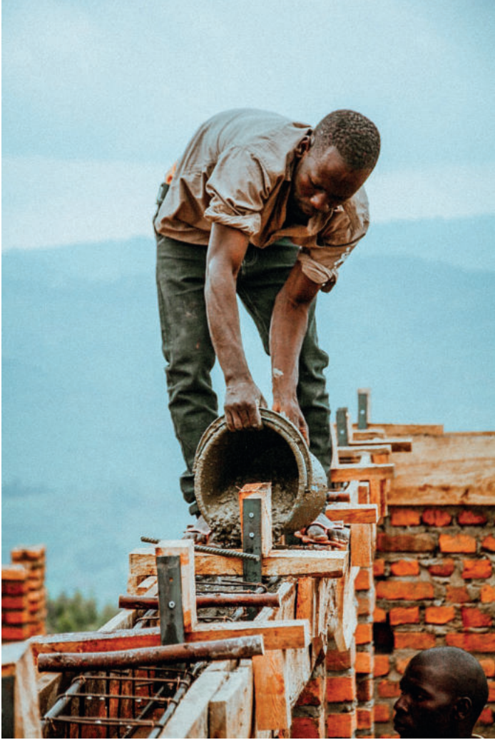
Ringanker betonieren Concreting the ring beam
