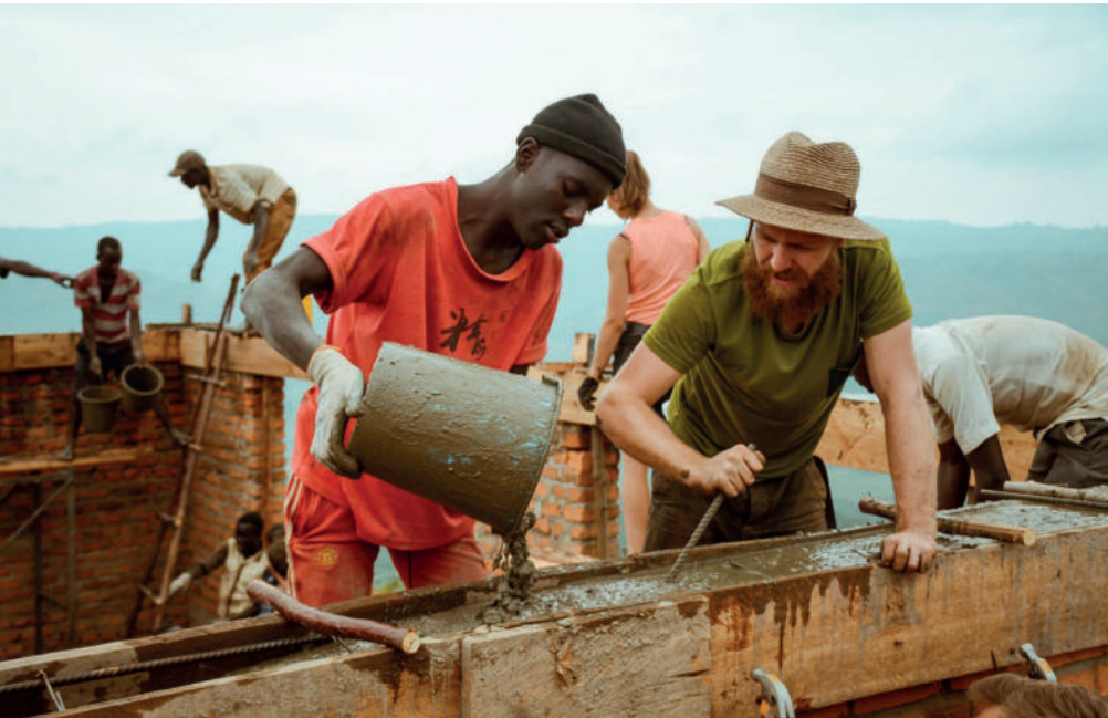
Ringanker betonieren Concreting the ring beam
