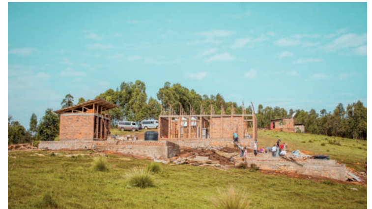
Konstruktion: Fundament, Ziegelmauer, Beton-Ringanker, Dachbinder Construction: foundation, brick wall, concrete ring beam, roof trusses
