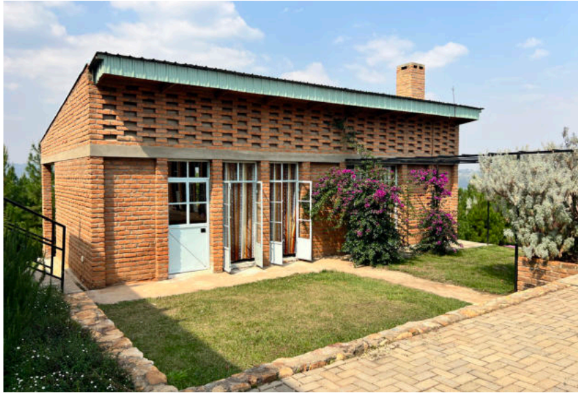
Lerncluster Construction of the foundations for farmer Salongo's new building
