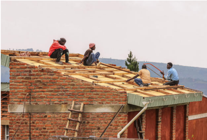
Reparaturen am Dach repair works on the roof
