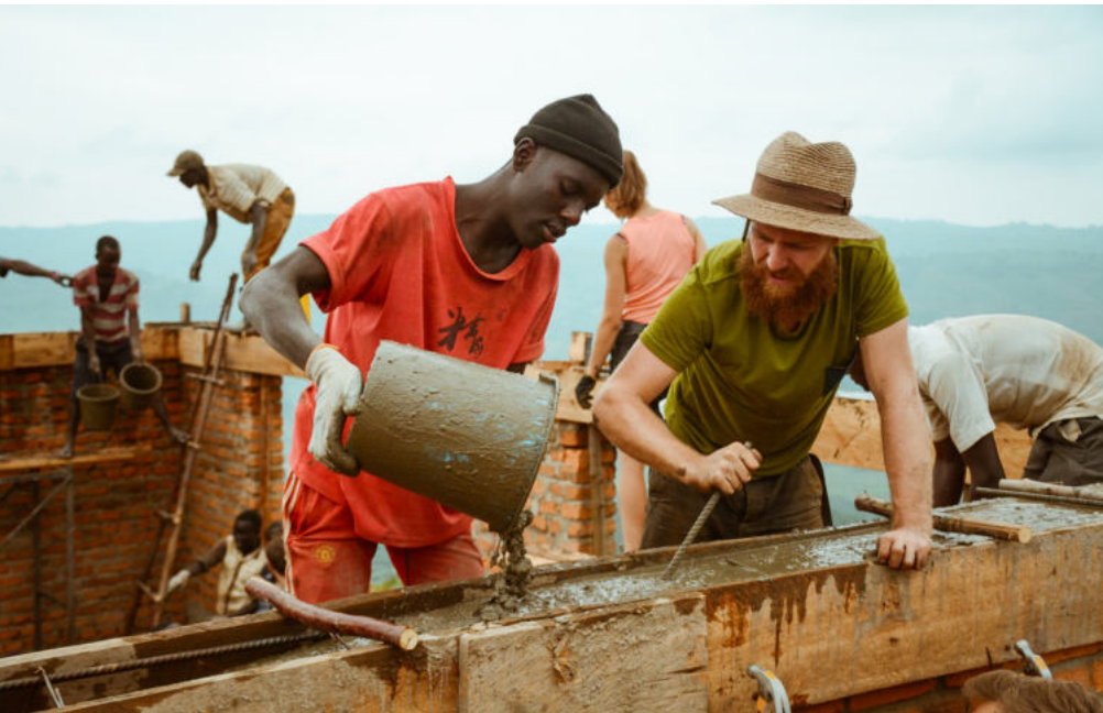
Ringanker betonieren Concreting the ring beam
