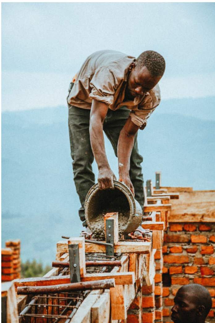
Ringanker betonieren Concreting the ring beam
