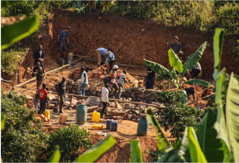
Bau der Fundamente des Neubaus für den Farmer Salongo Construction of the foundations for farmer Salongo's new building
