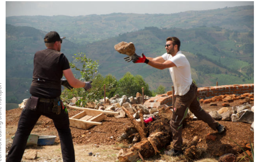
Teamwork beim Steintransport Teamwork during stone transport
